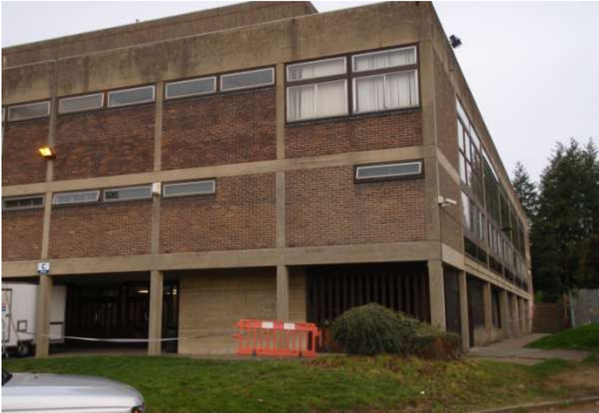
Plate 3 Block C- to be demolished (looking west)
