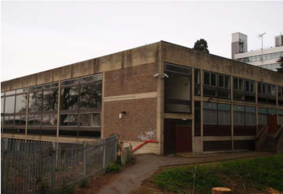
Plate 9 Looking at Block C at north corner
