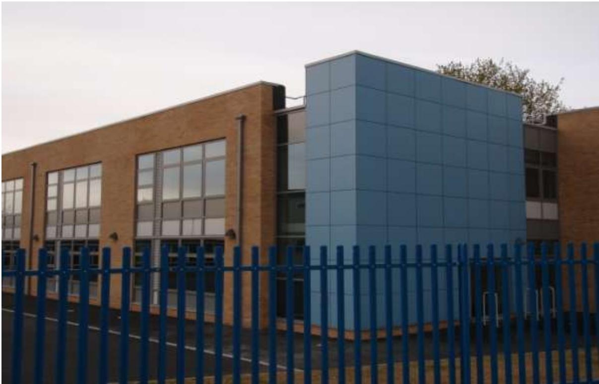
Plate 1 Buildings of Mid Kent College (looking south, see Figure 24).
