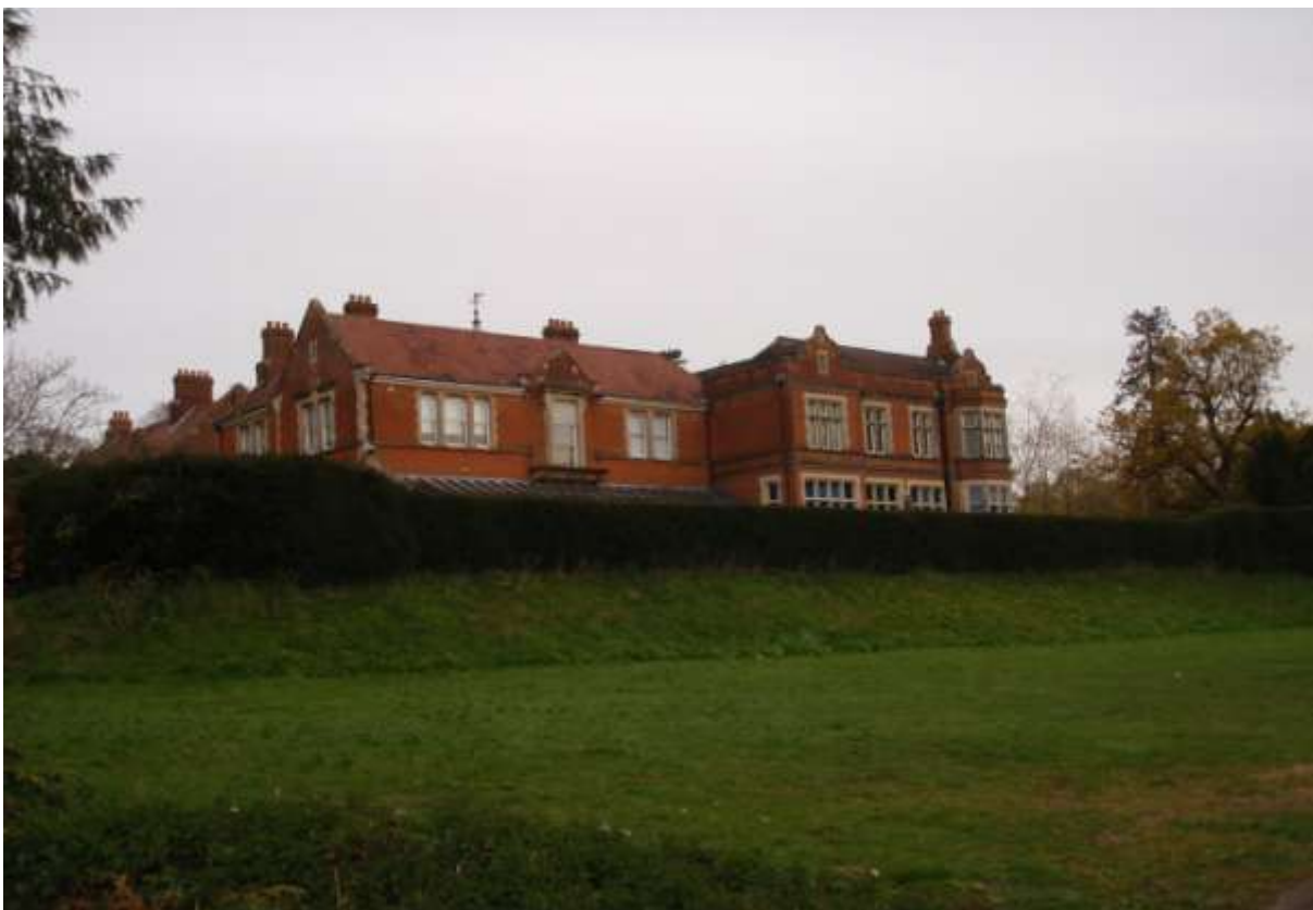
Plate 8. Looking north at Oakwood House
