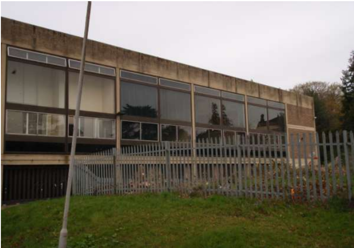
Plate 6 Block C (looking west)
