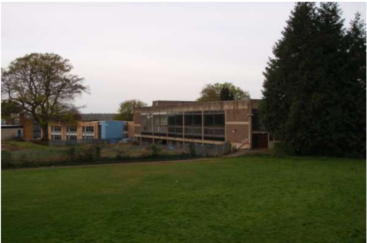
Plate 14 Looking south from centre of PDA
